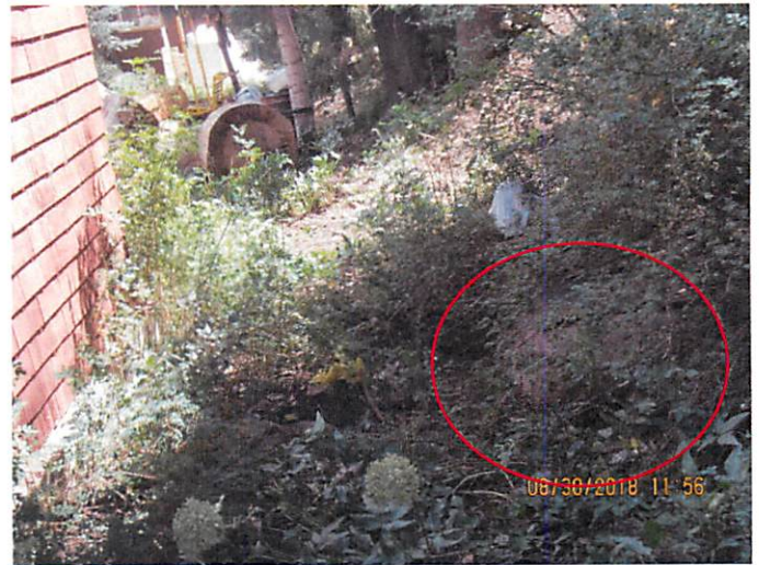
Photo 4: Location of Cesspool (outlined) on 4711 Aspen Ave
