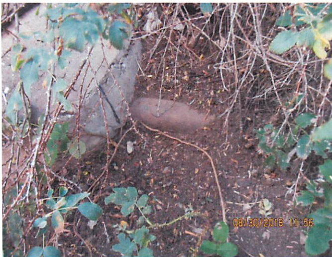
Photo 3: Sewer Line from 4721 Aspen Entering Community Cesspool located at 4711 Aspen Ave
