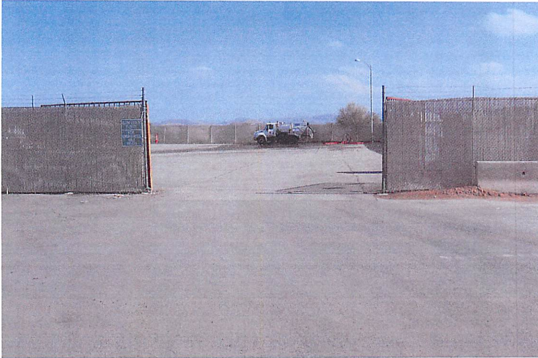
Street View of Main entrance of facility
