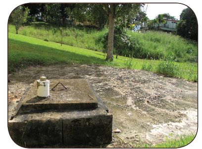
Keep septic tanks sealed.
