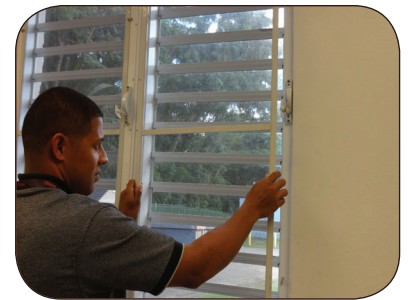
Install or repair window & door screens.
