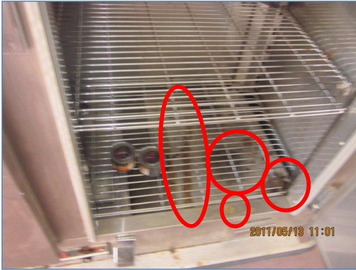
A1e. Hot holding units with debris left inside. All equipment must be properly cleaned.
