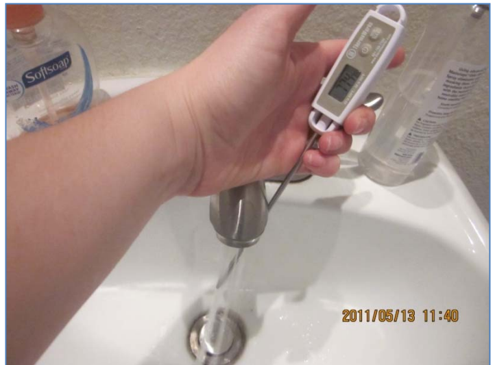
A2d. Hot water in bathroom sink reached only 77.4°F. Regulations require all handsinks to reach 100°F rapidly.
