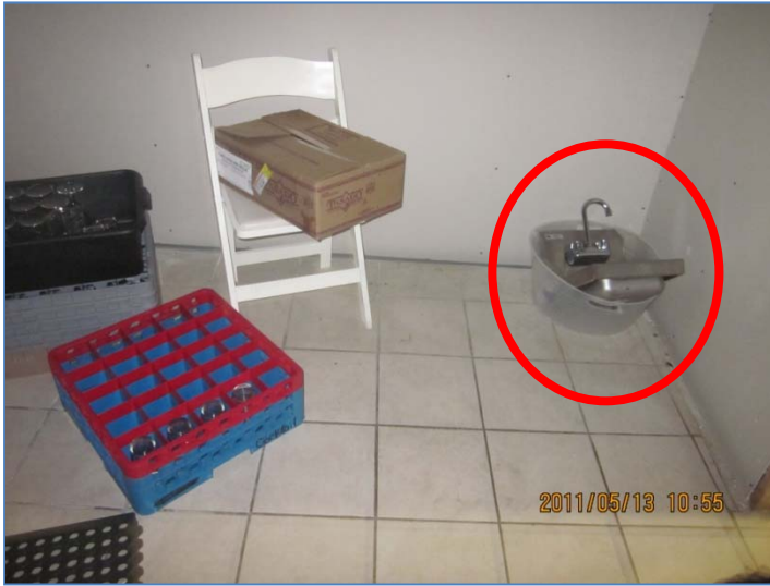
A2a. Sole handsink in kitchen is not installed.
