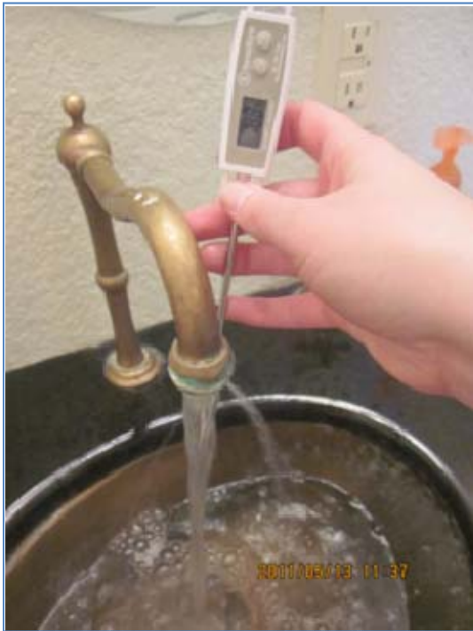
A2c. Hot water in bathroom sink reached only 78.8°F. Regulations require all handsinks to reach 100°F rapidly.
