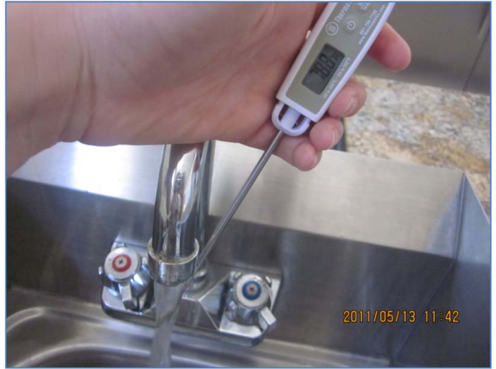
A2b. Handsink in bar only reached 78.8°F. Regulations require all handsinks to reach 100°F rapidly.
