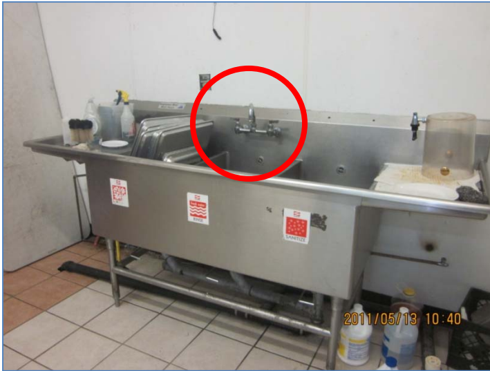
A1a. Three compartment sink: faucet neck does not reach all three compartments.
