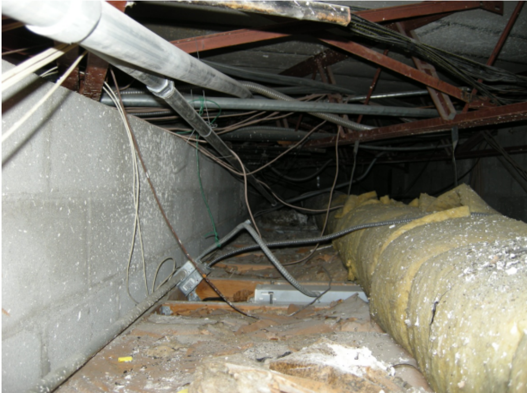
Photo 24 – Interior wall without attachment at the top of the wall.
