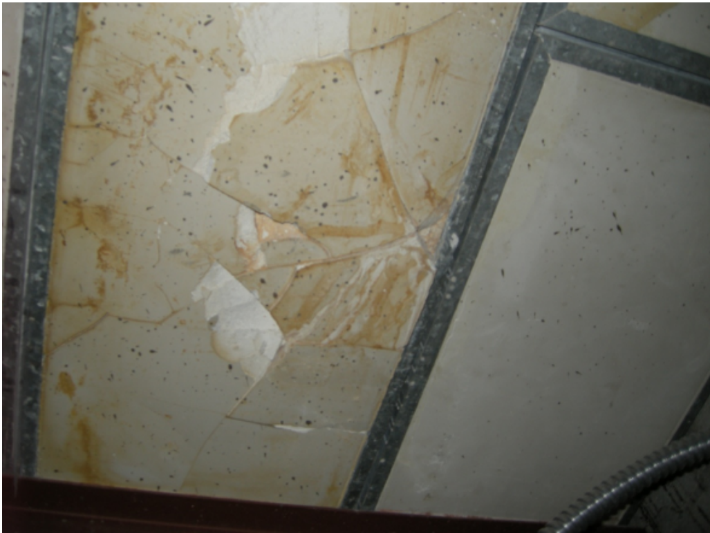
Photo 16 – Fractured gypsum roof panel.
