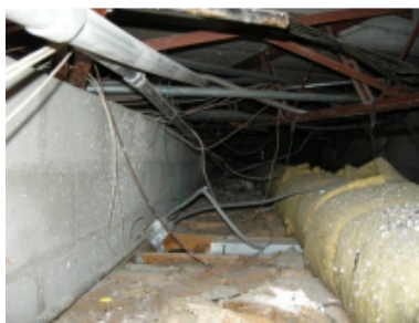
Photo 23 – Interior wall without attachment at the top of the wall.
