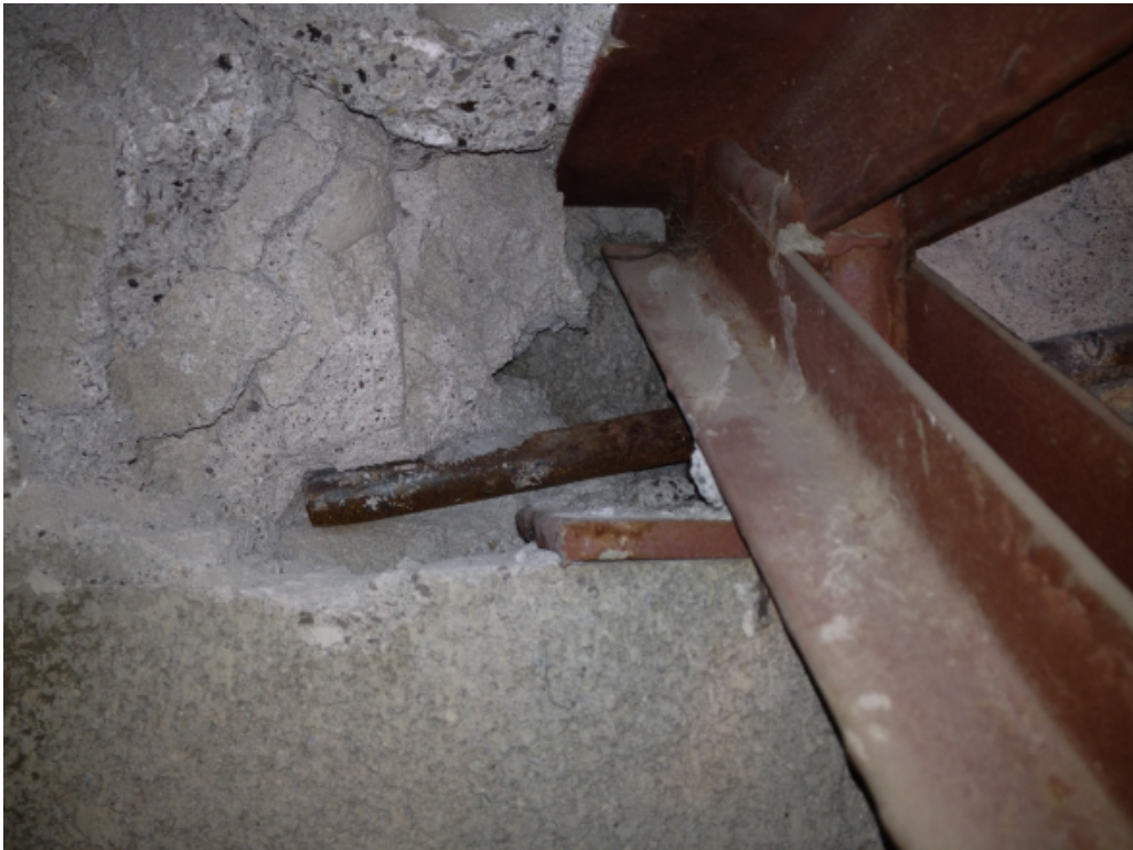
Photo 7 – Close up of the joist seat.
