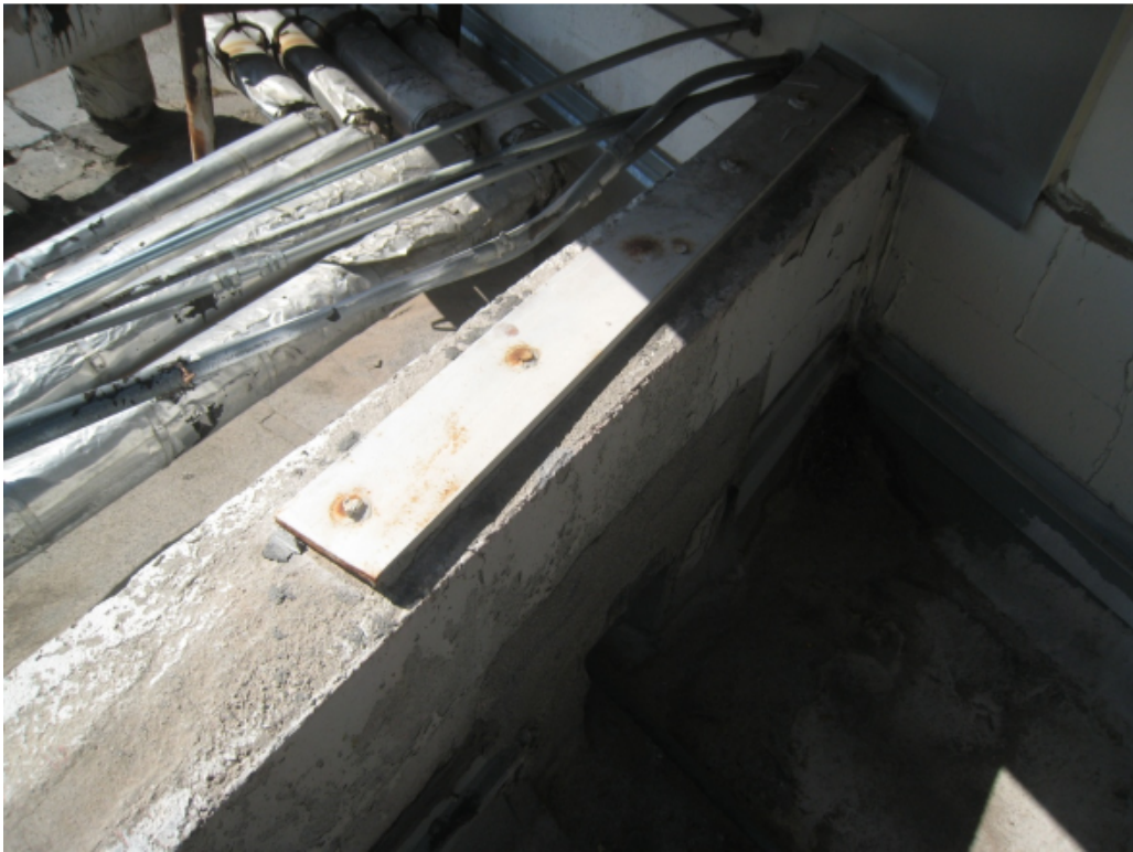
Photo 32 – Corroded lateral attachment.
