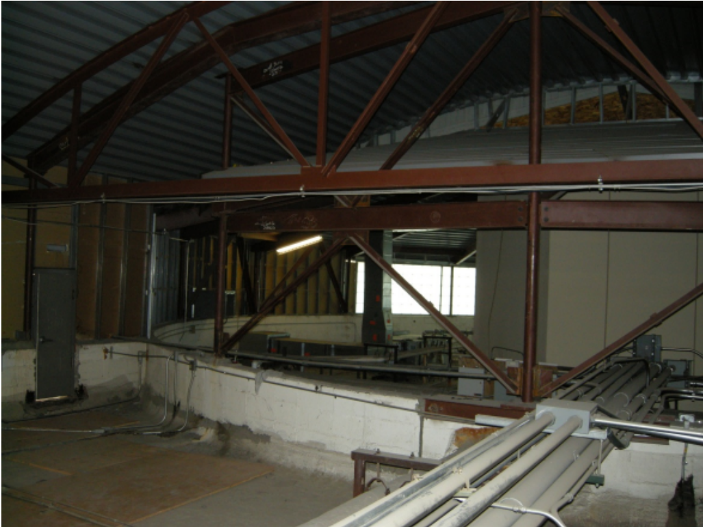
Photo 4 – Underneath over-framed roof
