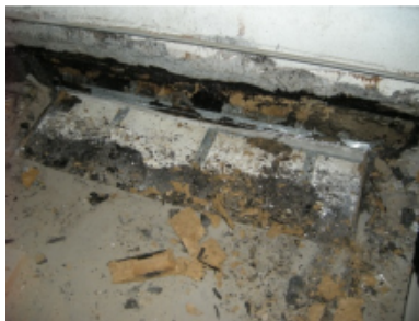
Photo 9 – Roof panels viewed from above with membrane removed.
