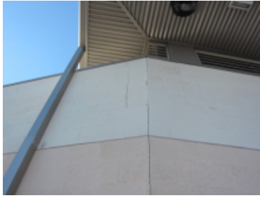
Photo 31 – Cracked at joint of intersecting walls.
