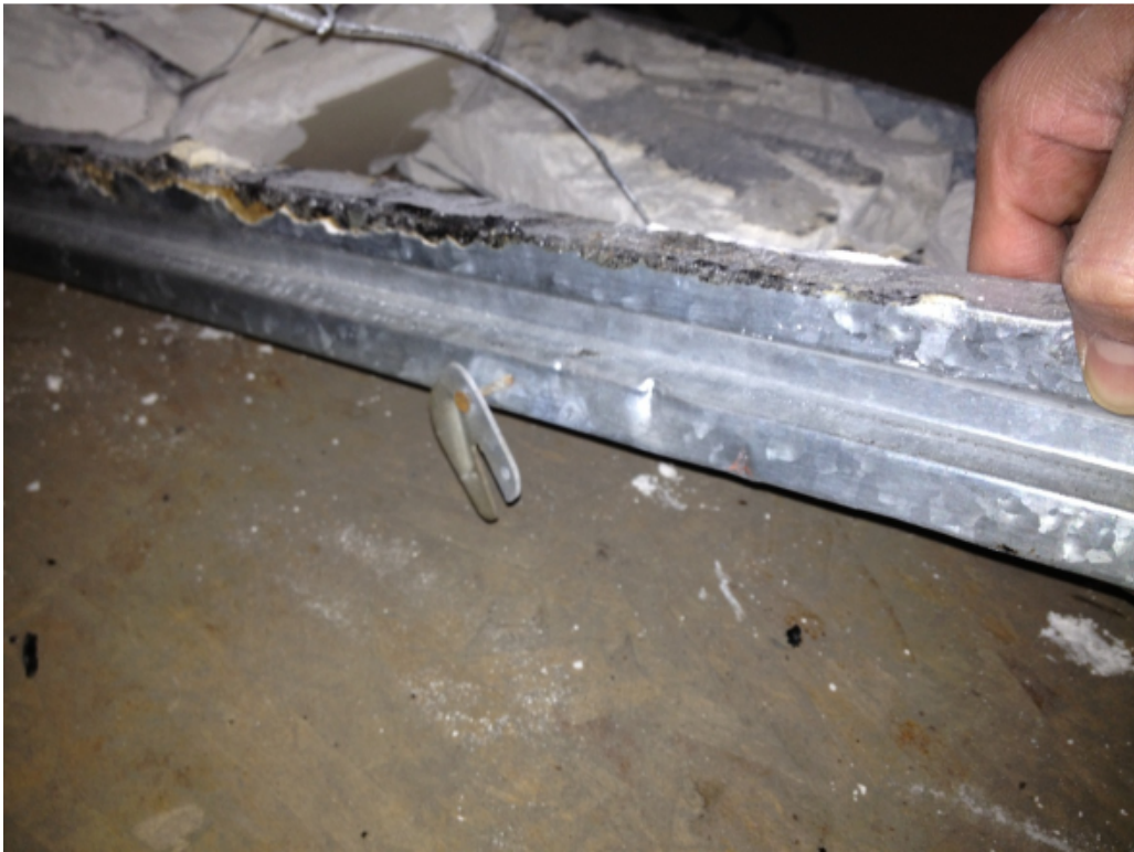
Photo 12 – A section of metal edged roof panel with attachment clip.
