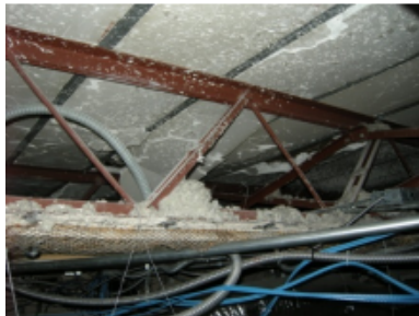
Photo 20 – Failed roof panel.
