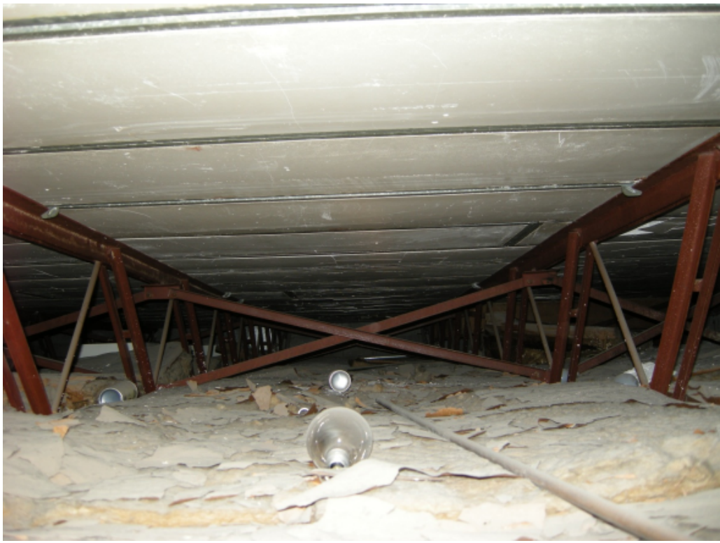
Photo 3 – Gypsum Panel Roof
