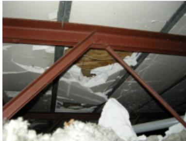
Photo 18 – Failed roof panel.
