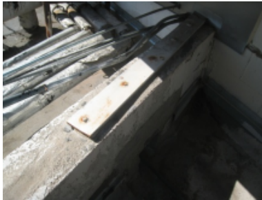
Photo 32 – Corroded lateral attachment.
