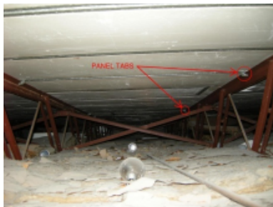
Photo 13 – Panel tabs located intermittently connecting the roof panels to the steel joists.
