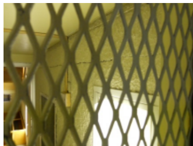
Photo 29 – Fracture on the interior side of an exterior wall.
