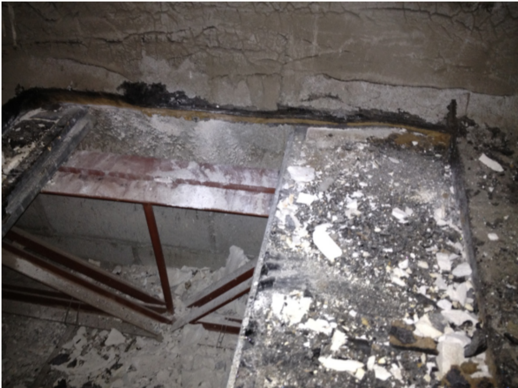
Photo 15 – Roof level with a panel section removed.
