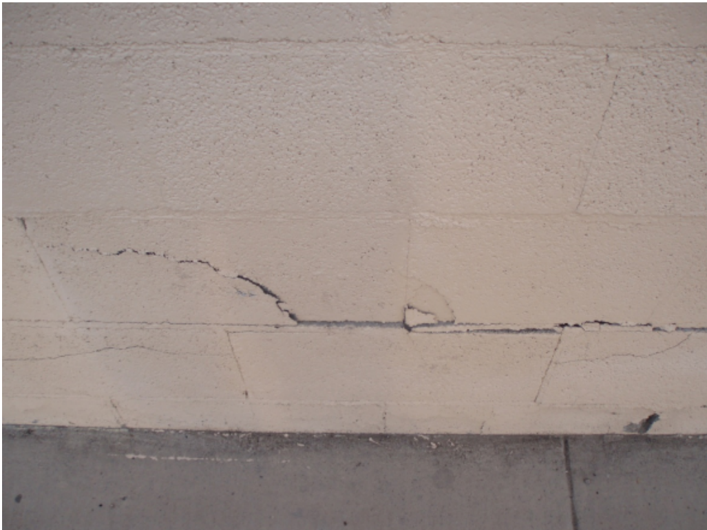
Photo 26 – Fracture at wall base.
