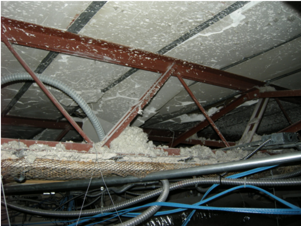
Photo 20 – Failed roof panel.
