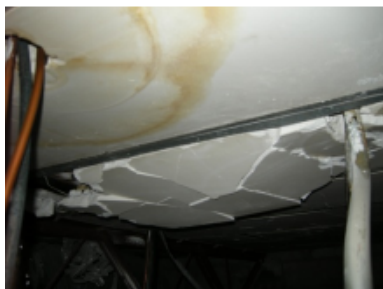
Photo 21 – Failed roof panel.
