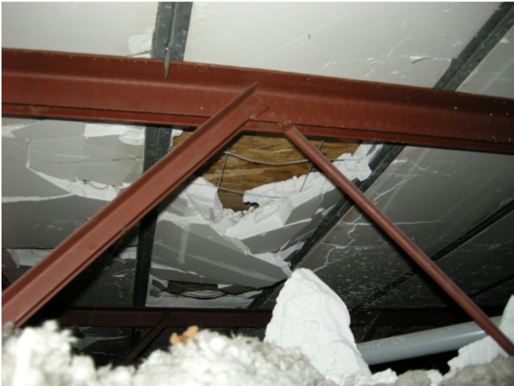
Photo 18 – Failed roof panel.
