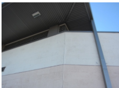
Photo 30 – Cracked formed at intersecting walls.
