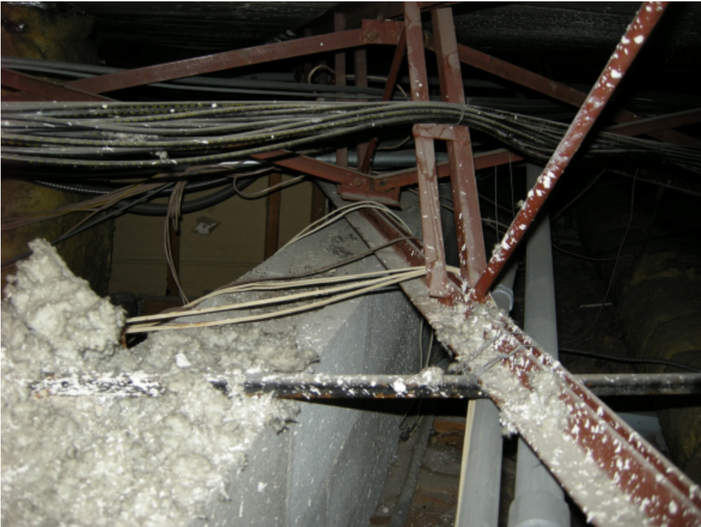
Photo 23 – Interior wall with no attachment at the top of the wall.
