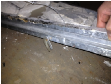
Photo 12 – A section of metal edged roof panel with attachment clip.
