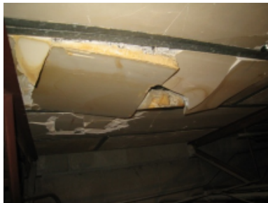
Photo 19 – Failed roof panel.
