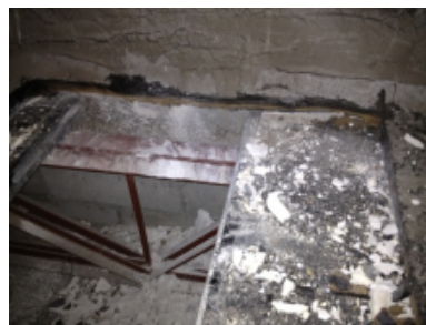
Photo 15 – Roof level with a panel
