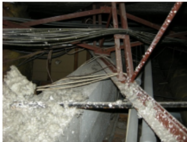
Photo 24 – Interior wall with no attachment at the top of the wall.
