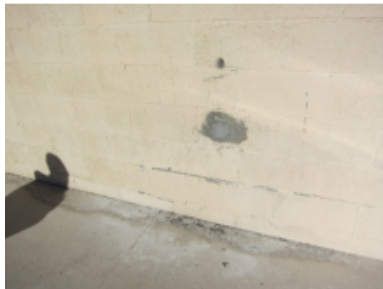
Photo 28 – Fracture at wall base.
