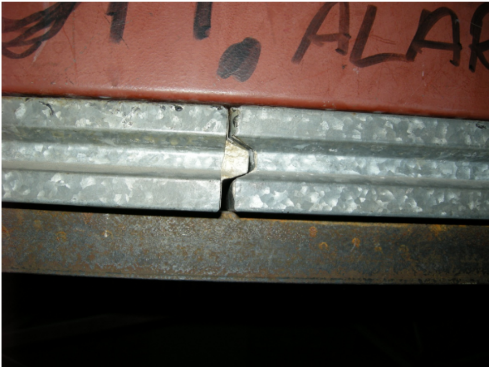
Photo 2 – Joint between Roof Panels
