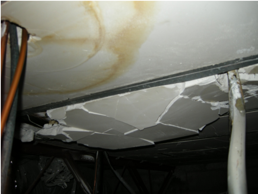
Photo 21 – Failed roof panel.
