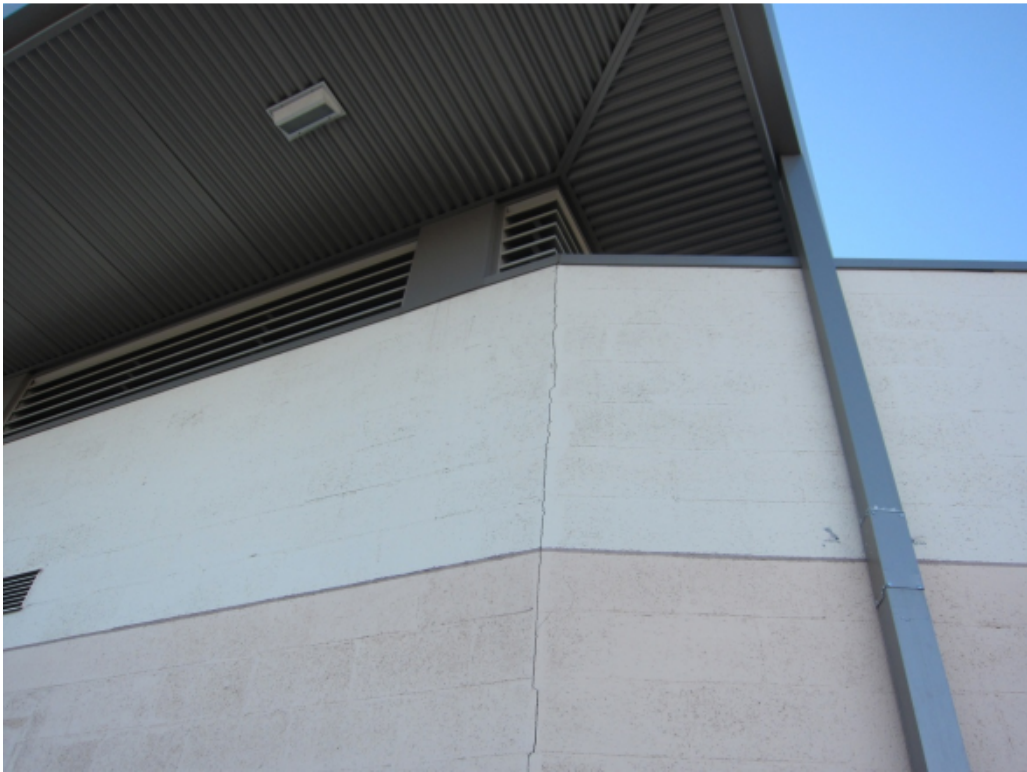
Photo 30 – Cracked formed at intersecting walls.
