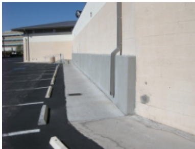
Photo 5 – Concrete buttress wall
