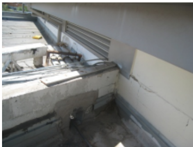
Photo 33 – Corroded lateral attachment.
