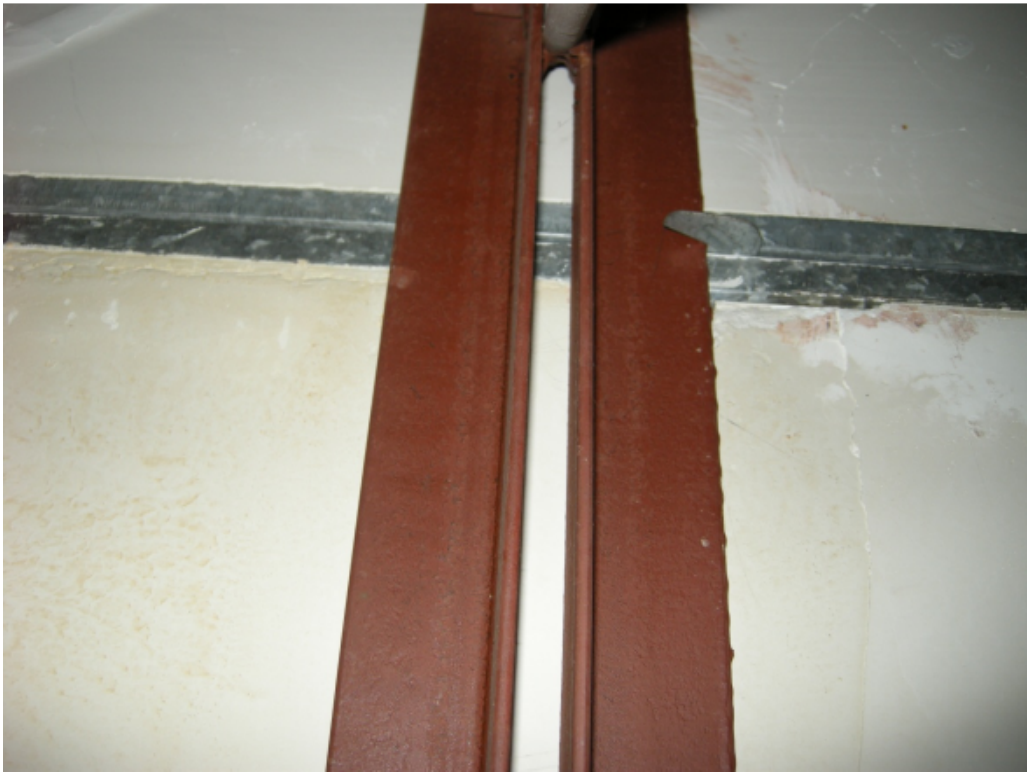
Photo 14 – Panel tab connection seen from below the joist top chord.
