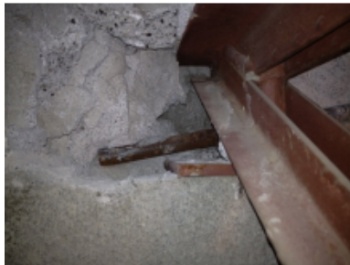
Photo 7 – Close up of the joist seat.
