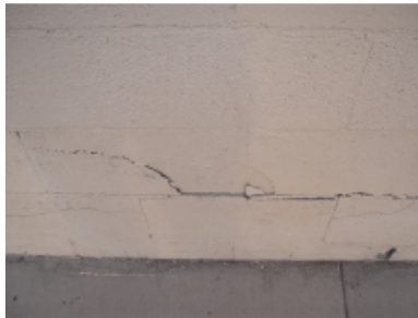
Photo 26 – Fracture at wall base.
