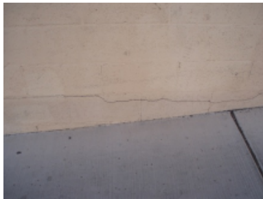
Photo 27 – Fracture at wall base.
