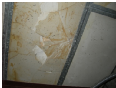
Photo 16 – Fractured gypsum roof panel.
