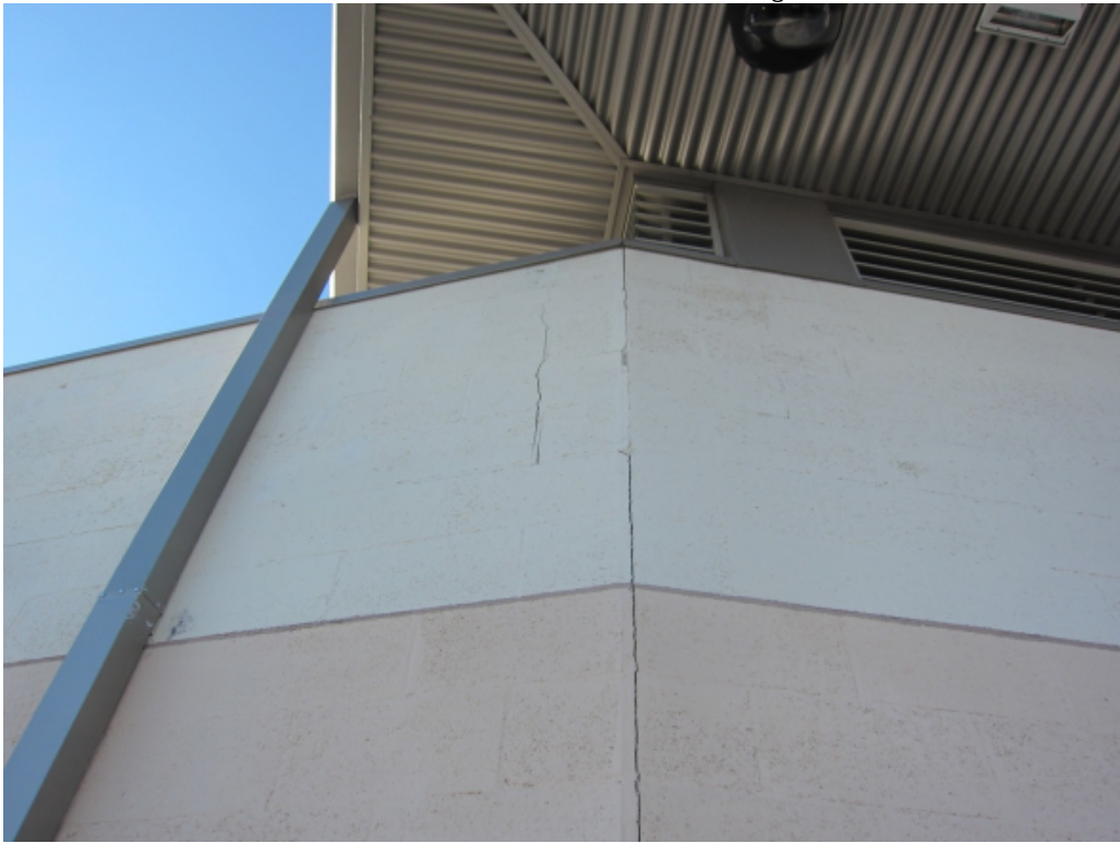
Photo 31 – Cracked at joint of intersecting walls.
