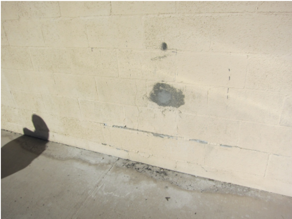
Photo 28 – Fracture at wall base.
