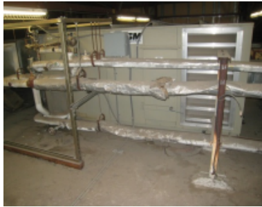
Photo 22 – Typical rooftop mechanical unit.
