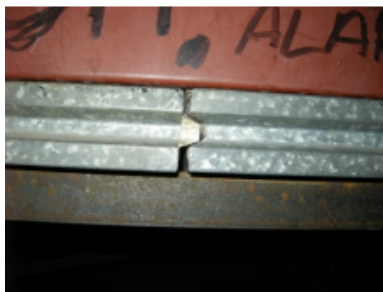
Photo 2 - Joint between Roof Panels
