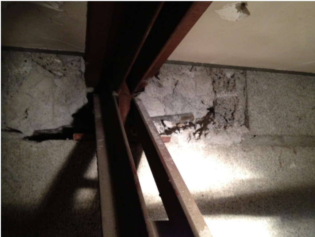
Photo 6 – Steel joist seat.
