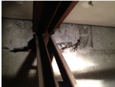
Photo 6 – Steel joist seat.
