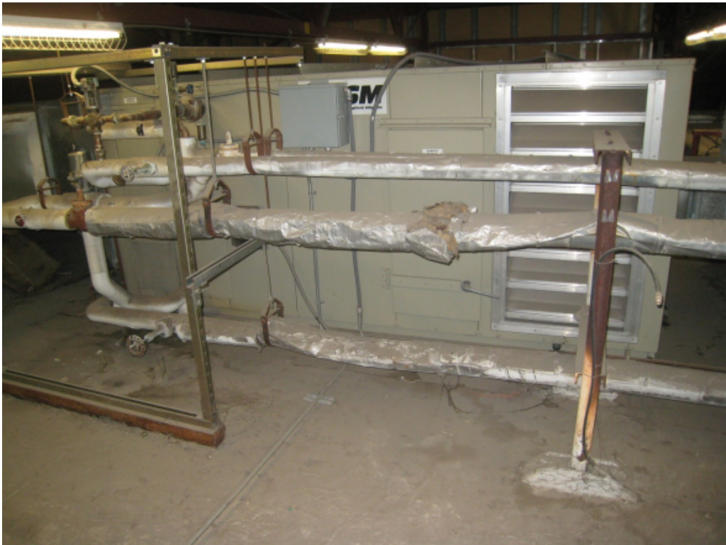
Photo 22 – Typical rooftop mechanical unit.
