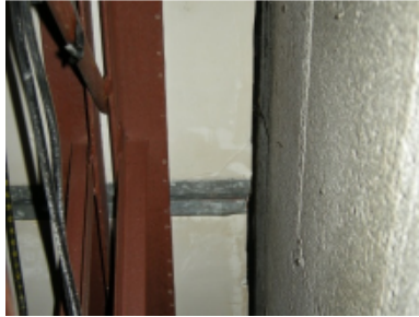
Photo 8 – Gap between the roof panels and the masonry wall.
