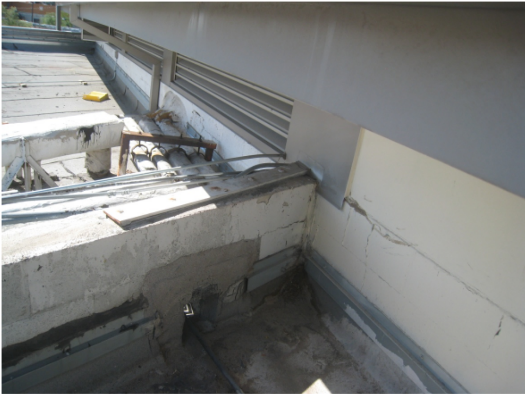
Photo 33 – Corroded lateral attachment.
