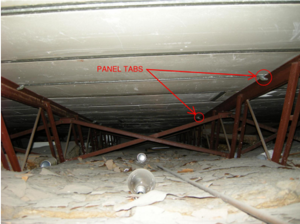
Photo 13 – Panel tabs located intermittently connecting the roof panels to the steel joists.
