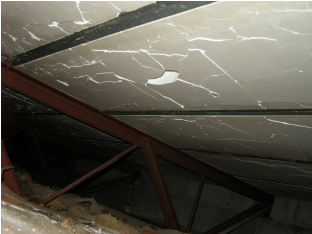
Photo 17 – Gypsum roof panels showing major fractures.
