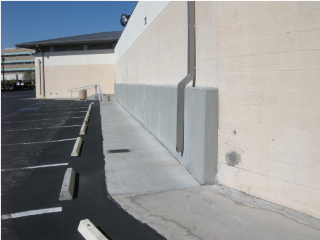
Photo 5 – Concrete buttress wall
