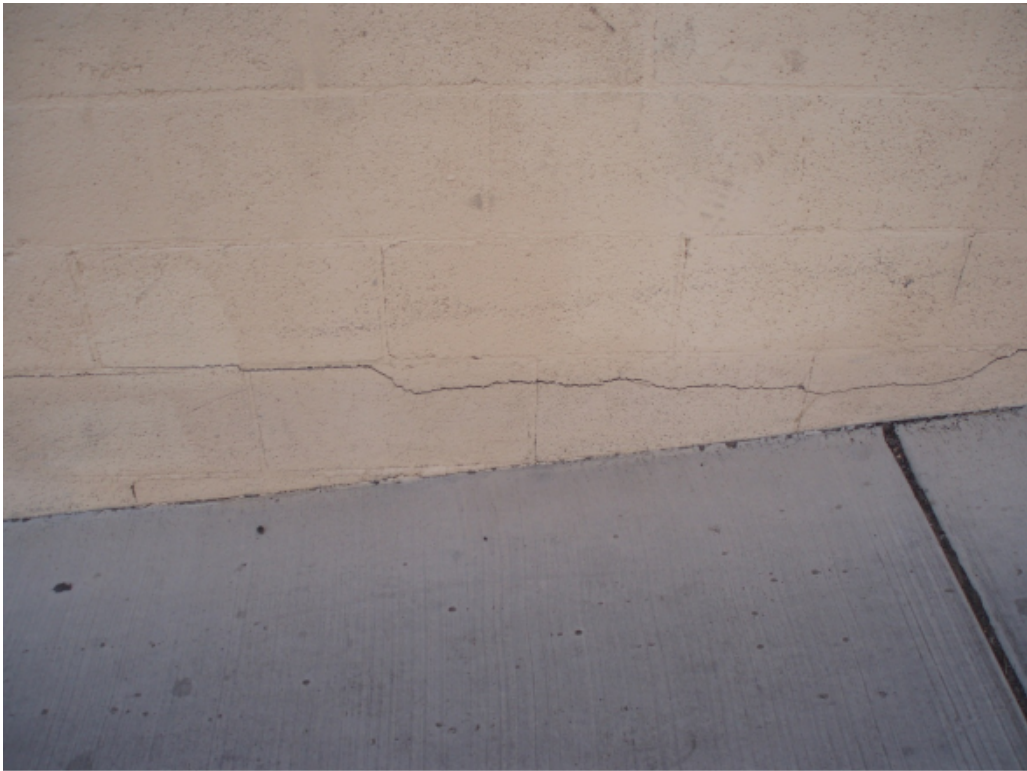
Photo 27 – Fracture at wall base.
