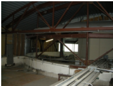
Photo 4 – Underneath over-framed roof
