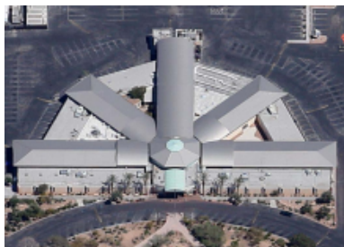
Photo 1 - PHC Main Building Aerial View
