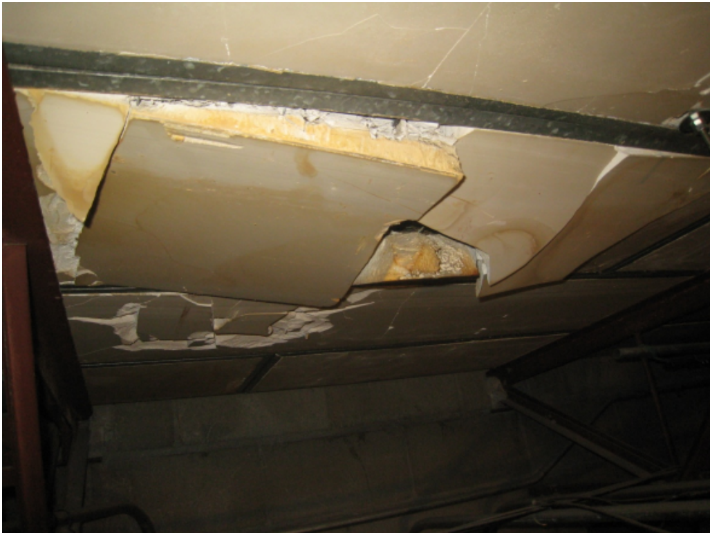
Photo 19 – Failed roof panel.
