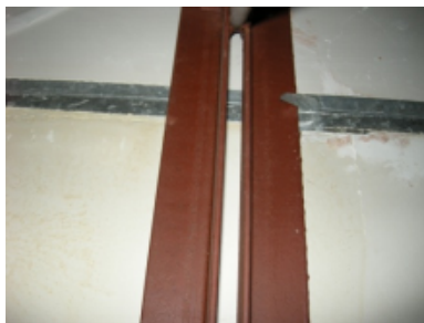
Photo 14 – Panel tab connection seen from below the joist top chord.
