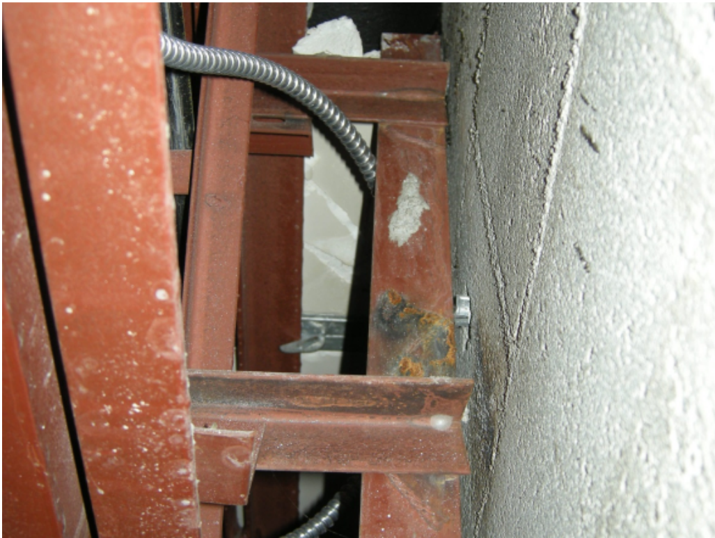
Photo 10 – Joist bridging anchor has separated from the masonry wall.
