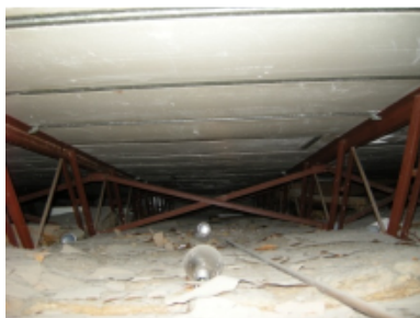
Photo 3 - Gypsum Panel Roof
