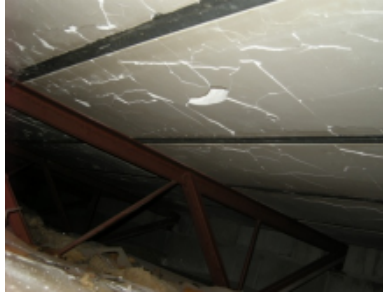
Photo 17 – Gypsum roof panels showing major fractures.
